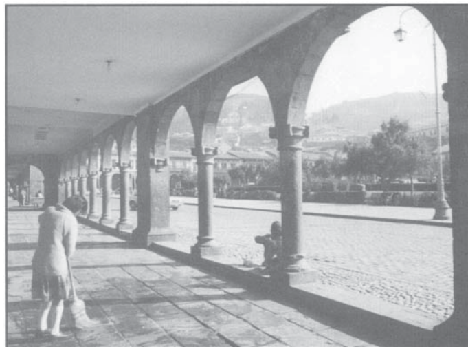
Fig. 1. Plaza de Armas, Cuzco, Peru. This central square acts as a huge courtyard, symbolizing the civic center.
